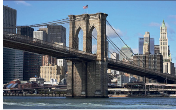
Brooklyn Bridge looking toward Manhattan
