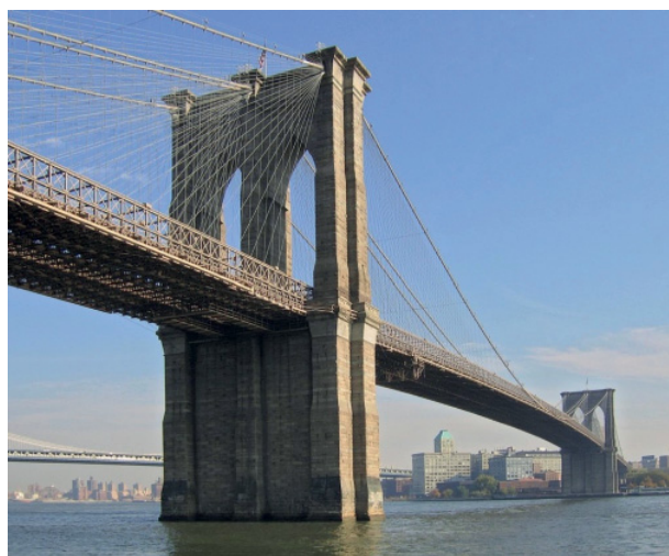
Bridge seen from Manhattan
