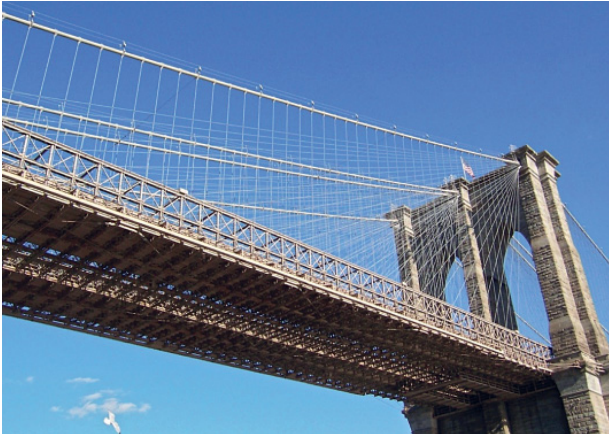
View of the bridge looking up at roadbed
