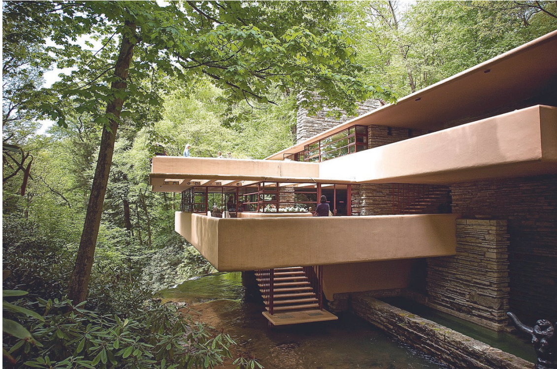
Fig. 17. Fallingwater, stair to stream [wikimedia]
